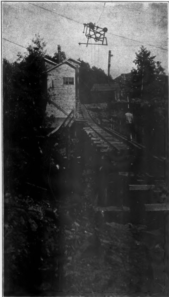
Tracks from Hoisting House to Slate Mill
